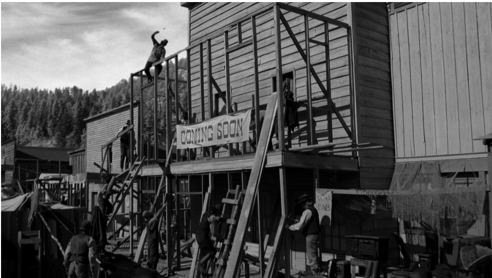
Deadwood under construction
